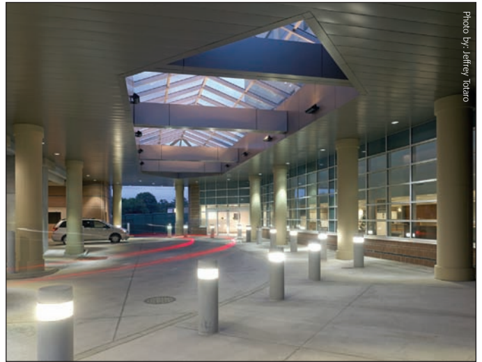
The entrance canopy provides protection from cold and inclement weather for patients and visitors as they move between the new garage and newly expanded ED.
